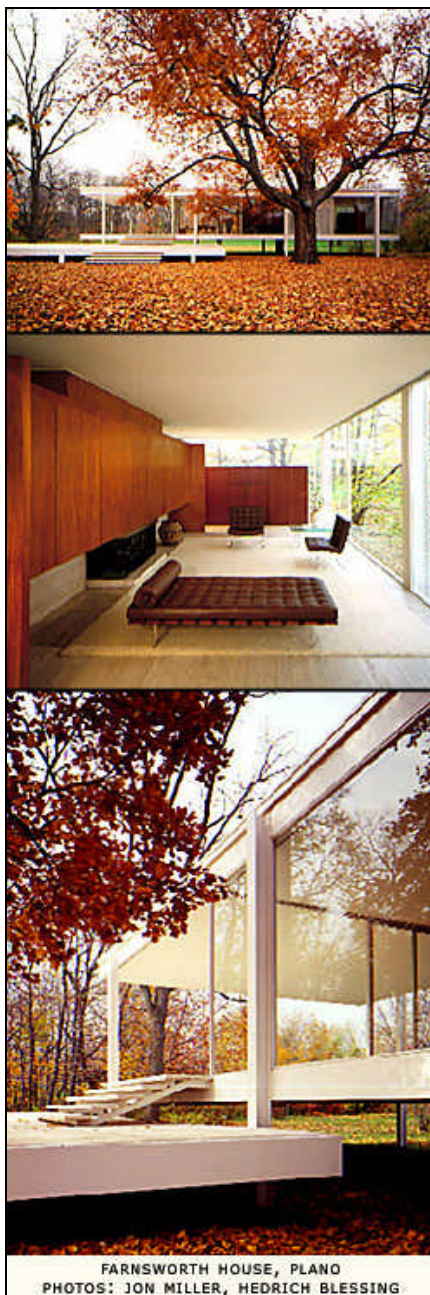
Farnsworth House, Plano, IL, photo by Jon Miller, Hedrich Blessing
