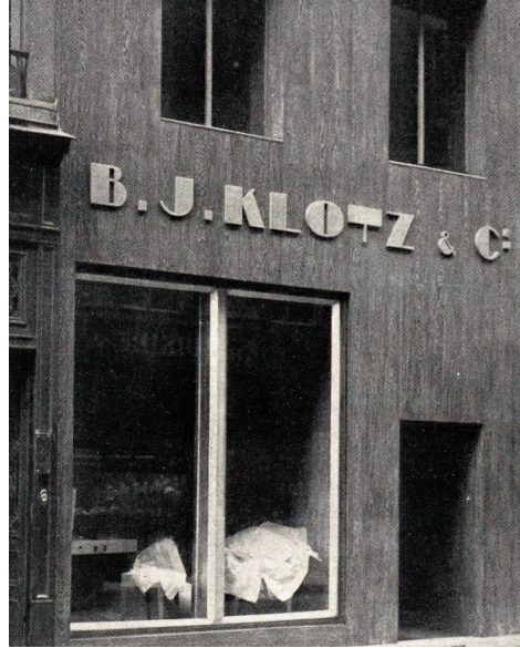
Fig. 3. B. J. Klotz, 3 Rue Miromesnil, Paris, France. Planar surfaces and large graphic signs were features of modern storefronts. Traditional stone materials were utilized, but innovative new products such as structural glass and porcelain-enamel panels made this architectural style easier to install. Architectural Forum , June 1929.
