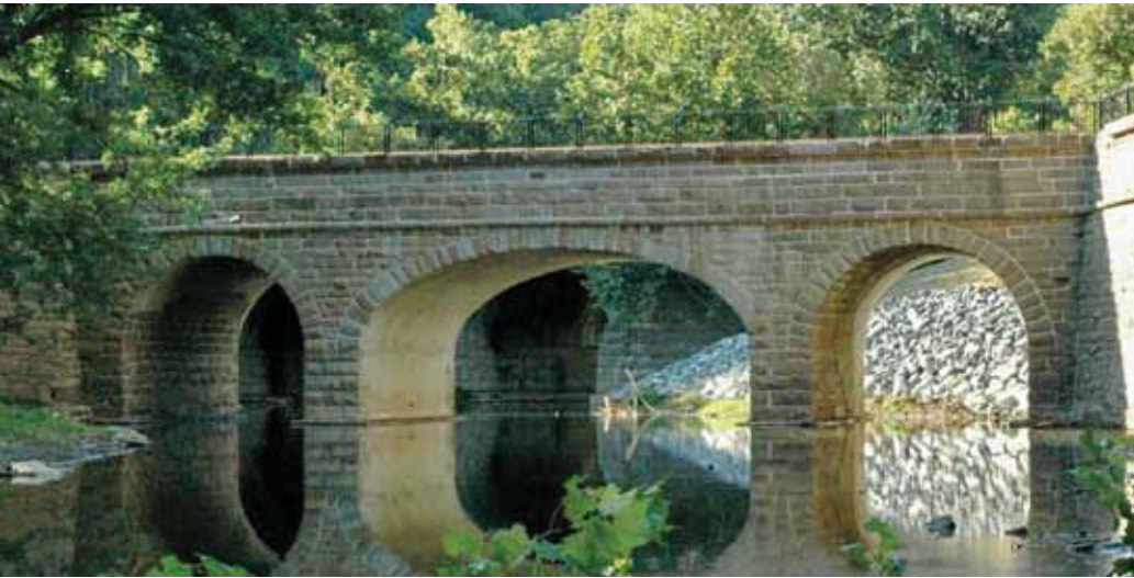
Fig. 11. Catoctin aqueduct after rehabilitation was completed, 2011. Photograph by George E. Lewis, Jr.
