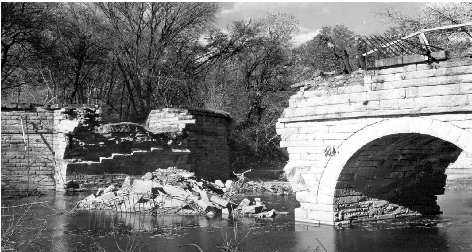
Fig. 1. Catoclin aqueduct, Lander, Maryland, collapsed center and western arches, 1973. The berm parapet and upstream spandrel wall had failed earlier. Note the railings bent in downstream direction, indicating predominate flood effects coming from tributaries and not the adjacent Potomac River. Courtesy of the C&O Canal National Historical Park Archives.
