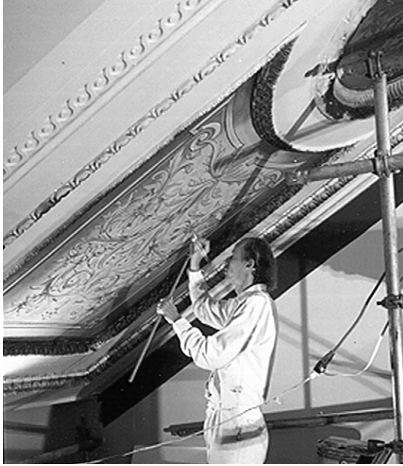
Fig. 6 Mock-up samples of work are important to reach team understanding and set a level of expectation for the final restoration product. In this case, lighting, surface texture, amount of glazes, and craft technique were all addressed in the mock-up sample. Photograph by Dietrich Floeter.
