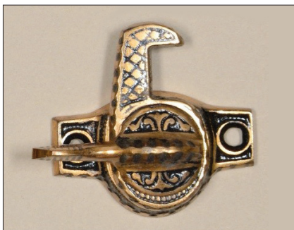
Fig. 7. Hobart B. Ives, double-action-cam sash fastener, ca. 1885. It uses an internal cam to operate an arm to first hook the keeper and then draw the two sash together. Photographs by author.
