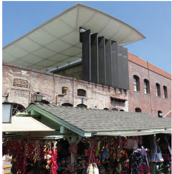
Fig. 6. View of the canopy shelter from Olvera Street, showing the vertical metal louvers, which provide protection from sunlight directly hitting the mural at the two sides and allow for a partial view of the mural and shelter from the street. Photograph © J. Paul Getty Trust, 2018.
