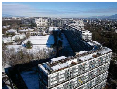
The Housing Complex of Lignon, George Addor, 1966. Geneva, Switzerland. Photo credit: Kyle Normandin
